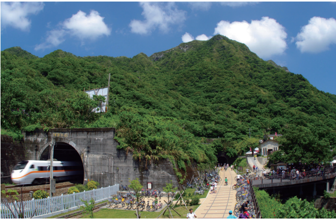
▲Figure 69 : Opening of Old Caoling Tunnel
